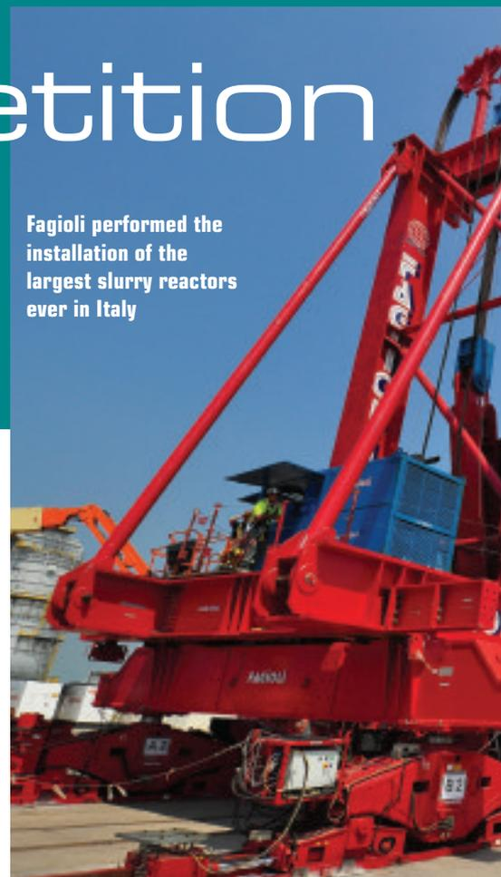
jacks, four skid shoes, an 80-meter high tower lift system utilizing four L600 strand jacks and a swivel system. Before the operation, Fagioli performed a test load of 2,400 tons in order to guarantee maximum safety.
